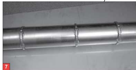
Insert slip joint assembly to complete connection
