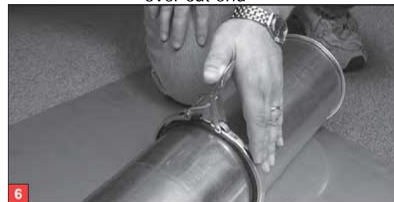
Adjust its length, snap clamp over O-ring and one end of the slip joint
