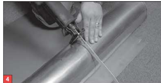
Cut pipe and remove any burrs
